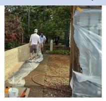
The Memorial Garden wall has a fresh look to it. Work began several weeks ago to re-point the grout in the wall. The old grout had deteriorated over time, allowing water to seep into the grout and promoting mold.
